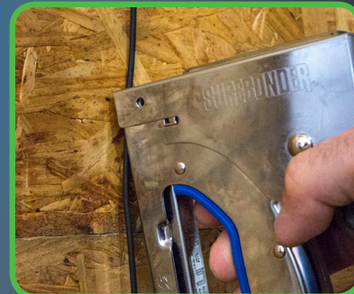
Secure 1 meter of cable with 20 staples on a wood panel
